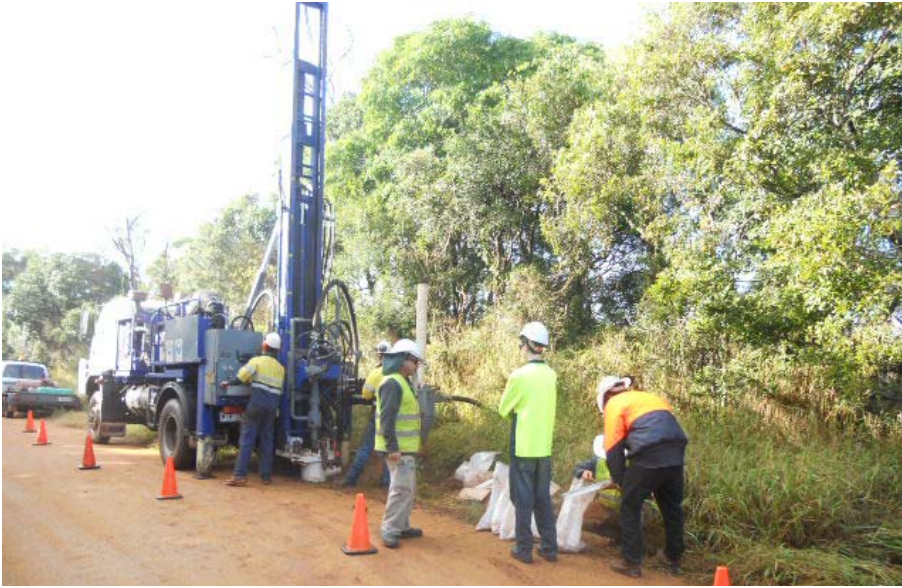
Figure 3: Underdale Drillers Carrying Out Roadside Drilling at Kingaroy Project
